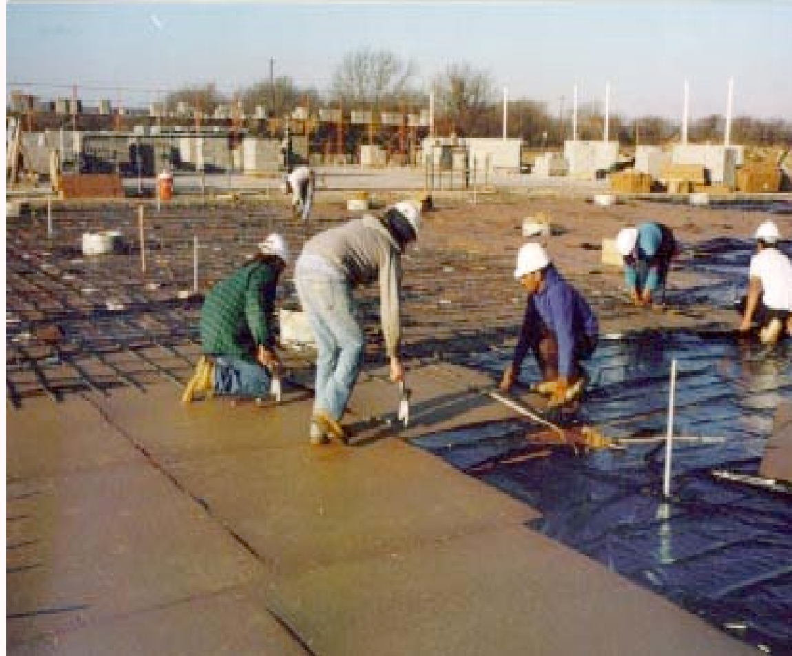
Placement of fiberboard coverings
