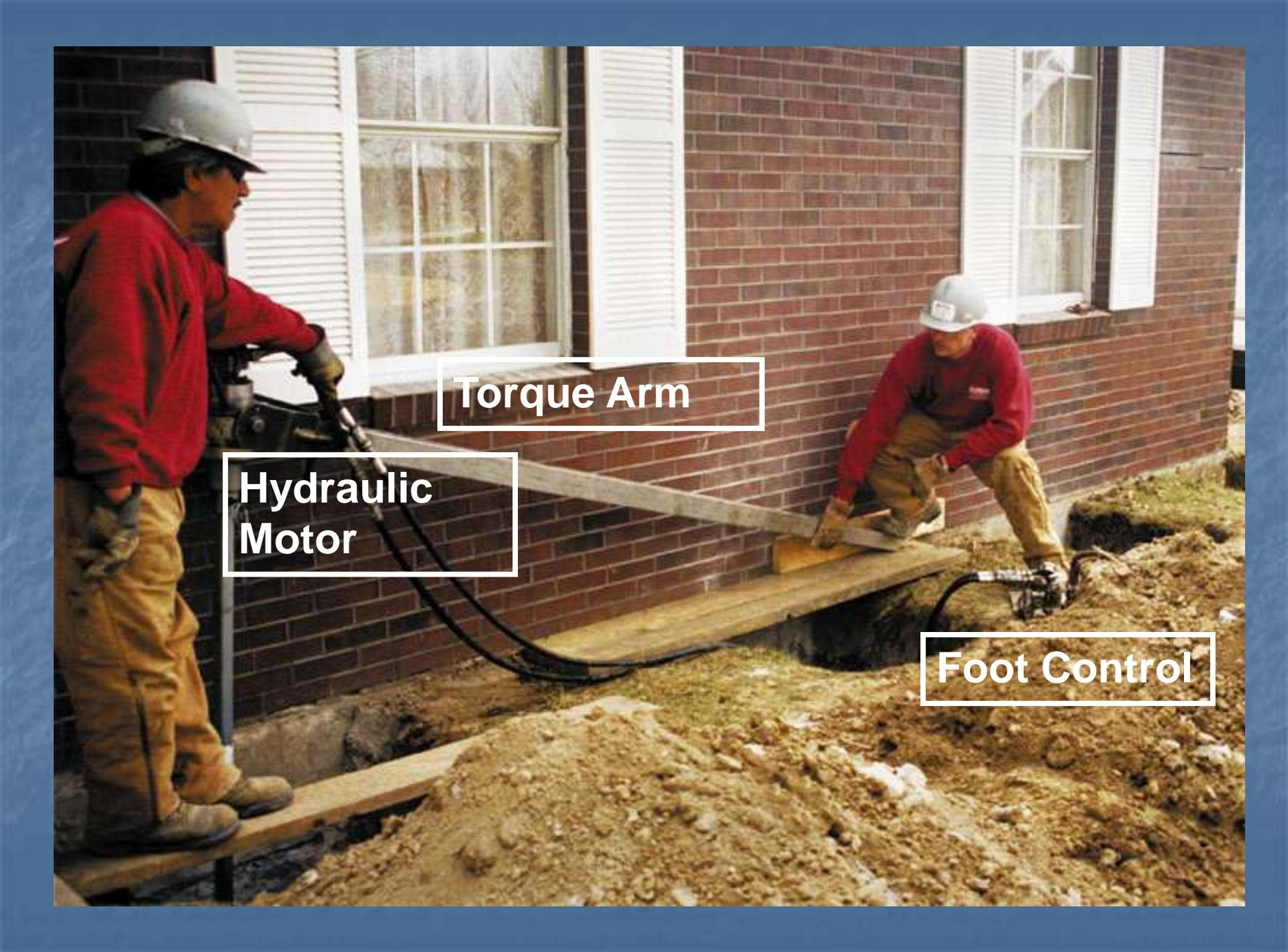
A construction worker in a red shirt and tan pants stands on a wooden plank, operating a hydraulic torque arm. The worker is wearing a grey hard hat and safety glasses. The torque arm is a long metal beam extending across a trench. A hydraulic motor is connected to the end of the torque arm. Another worker is kneeling on a wooden plank in the trench, operating the foot control. The background shows a brick building with windows and white shutters. The ground is dirt and gravel.
