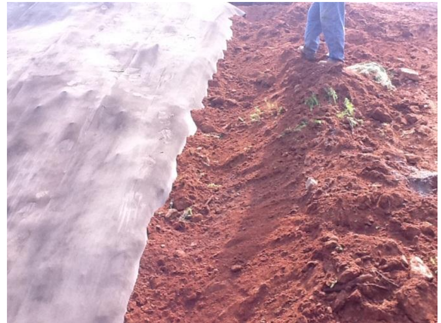
Right side anchoring of the Concrete Cloth
