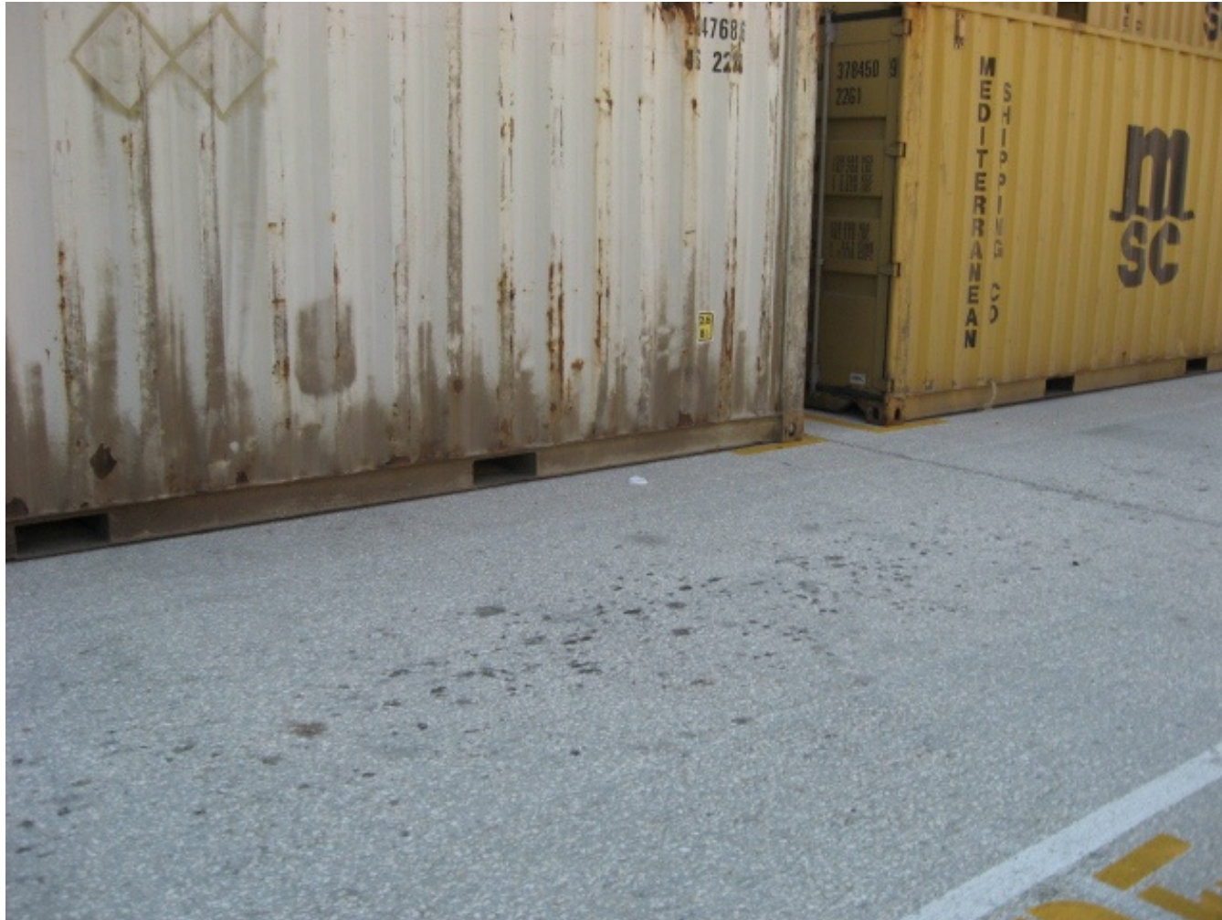
Point Loads from Container Corner Castings
