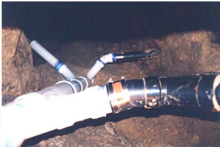
**Tunneling under slab for leak repair**
