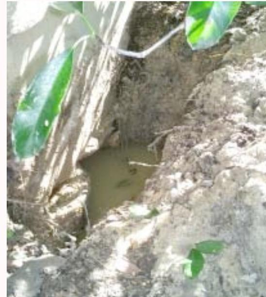
**Water ponding at grade beam / pier**
